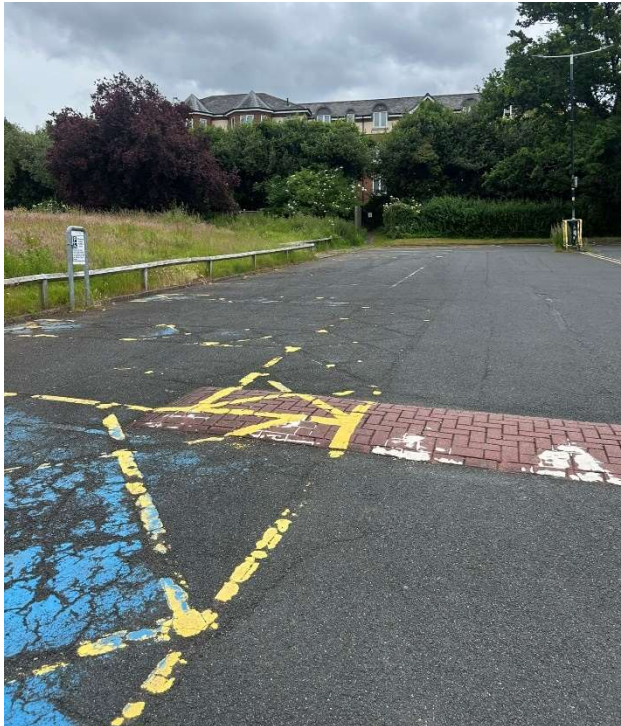
Photograph 4: School Drive Car park
